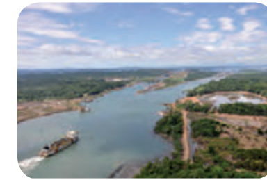
Dock deepening & extension
