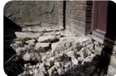
Lightweight concrete, standard concrete
