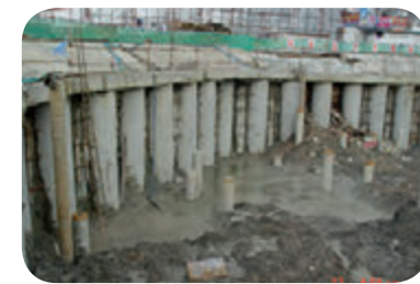
Foundation pile driving
