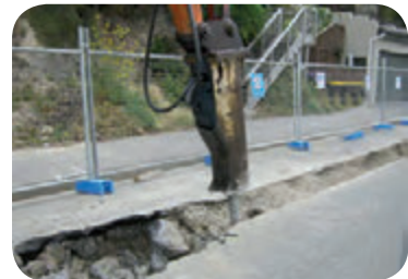
Trenching, pit building, ground excavation
