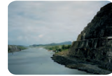
Canal deepening & extension
