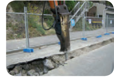
Trenching, pit building, ground excavation
