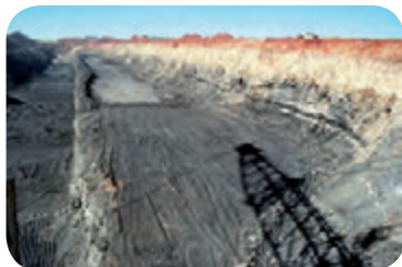
Overburden removal, bench, road & ramp levelling
